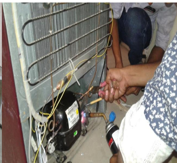
Fig5. Charging of Domestic Refrigerator
