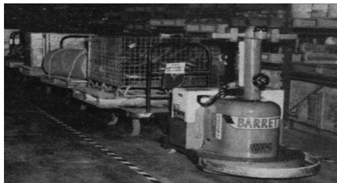
**Fig.1-First Automated Guided Vehicle(AGV) by Barret Electronics [1].**
